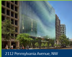
2112 Pennsylvania Avenue, NW
