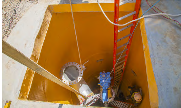
Picture 2. Wet well being installed.
