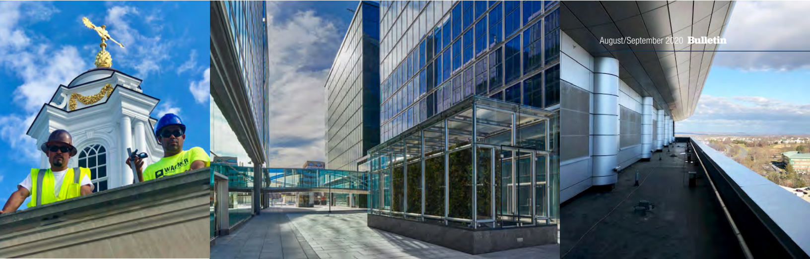
(Left to Right) Annapolis Post Office Restoration, Annapolis, MD – Wagner Roofing Company; Capitol Crossing, Washington, DC – Superior Ironworks, Inc.; INOVA Loudoun Phase 2B Patient Tower, Leesburg, VA – Kalkreuth Roofing and Sheet Metal, Inc.
