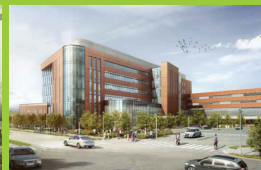
Virginia Hospital Center The Outpatient Pavilion and Garage
