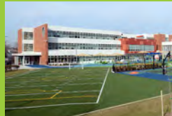
DC, Department of General Services Lawrence E. Boone Elementary School
