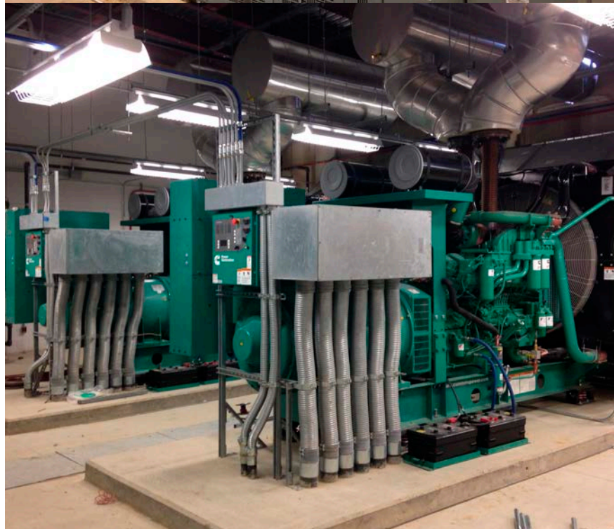
Ambulatory Care Center Phase I - Joint Base Andrews, Camp Springs, MD
