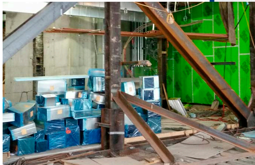
1785 Massachusetts Avenue NW Renovation, Washington, DC
