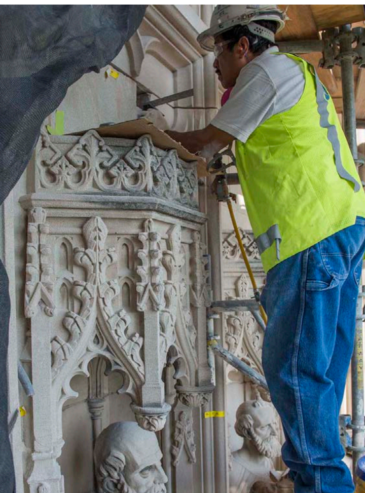
Top: 1275 Pennsylvania Avenue (Exterior Stone), Washington, DC
