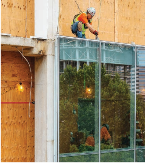
7900 Westpark Drive Renovation, McLean, VA
