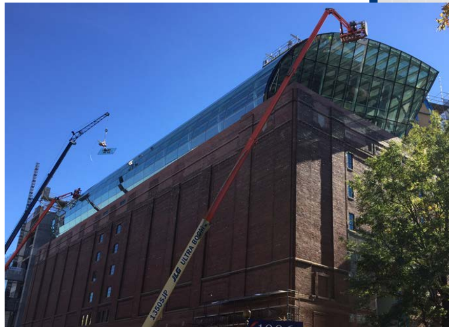
Doors & Windows: Exterior Glass Museum of the Bible, Washington, DC
