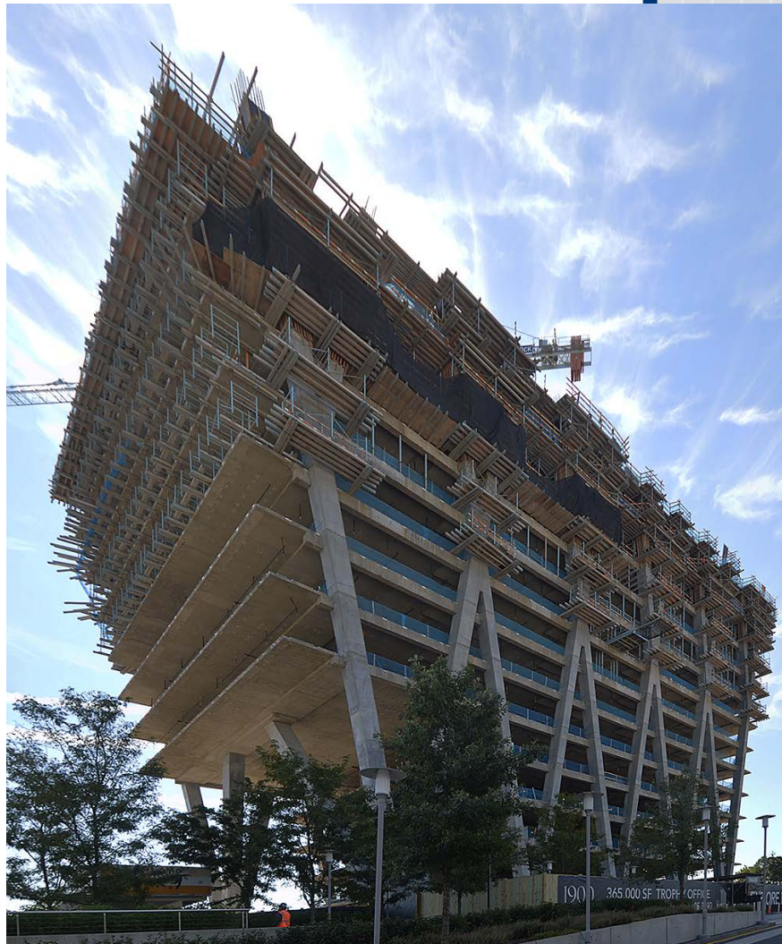
Concrete: Cast-in-place Concrete Reston Station Office Building 1, Reston, VA
