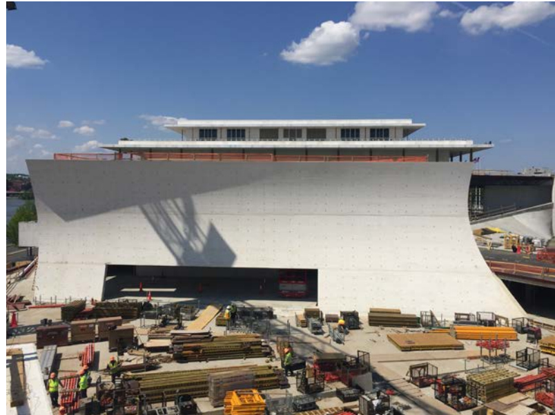
Kennedy Center Expansion, Washington, DC –The Lane Construction Corporation
