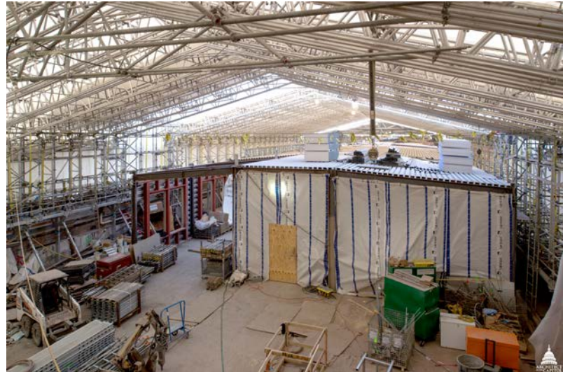
Cannon House Office Building - Phase 1 Renewal, Washington, DC – BrandSafway Services, LLC
