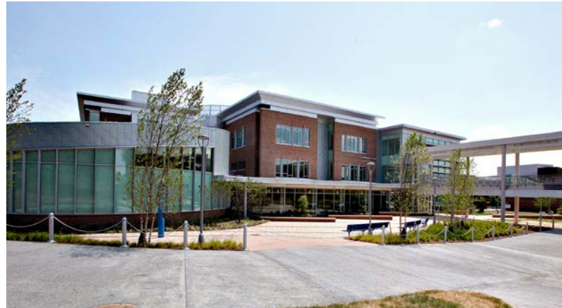
Prince George's Community College - Lanham Hall Renovation/Addition, Largo, MD – IronShore Contracting, LLC
