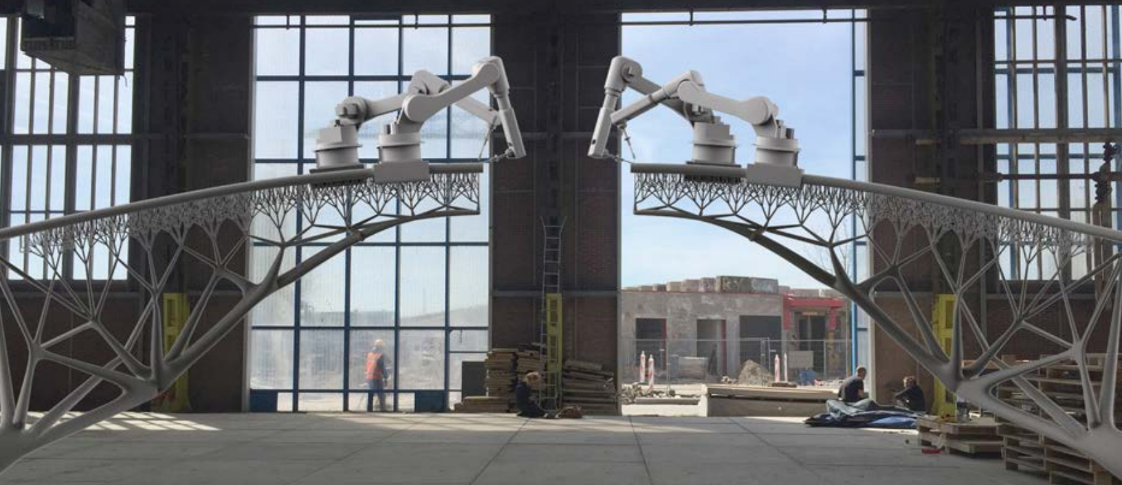
Producing the world's first 3D-printed bridge with robots "is just the beginning." https://www.dezeen.com/2015/12/30/video-interview-robots-worlds-first-3d-printed-bridge-mx3d-joris-laarman-movie/
