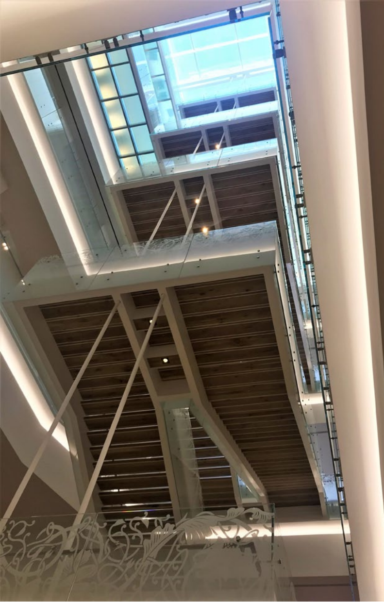
The grand stair, which appears to hang weightlessly from the 5th floor to the basement, forms the central spine of the museum.
