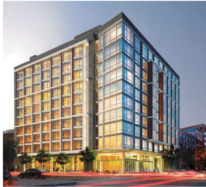
Turner Construction Company is building the 238-Room LEED Silver Hilton Garden Inn – M Street in Washington, DC
