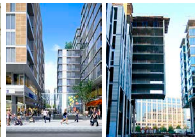
City Center DC – Cast-in-Place Concrete
