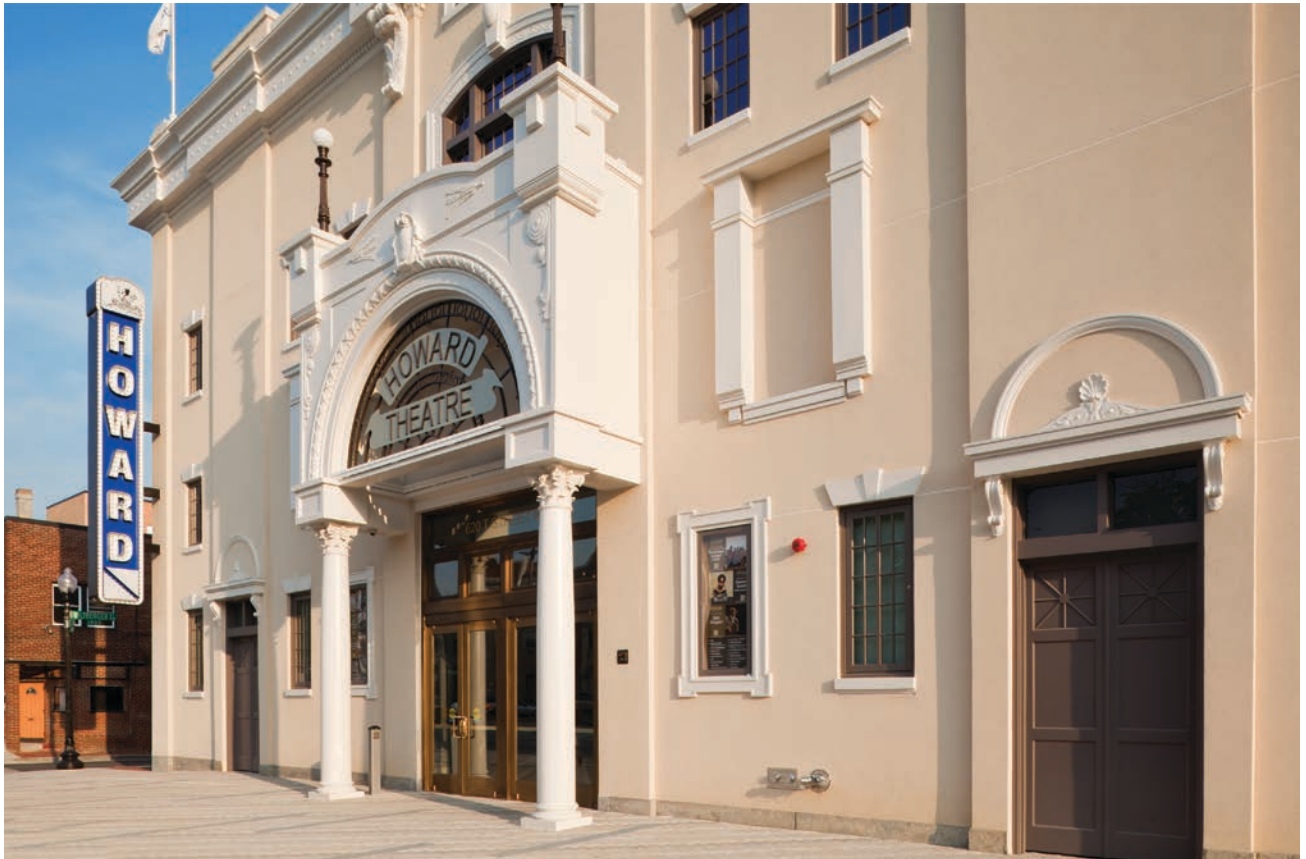
Howard Theatre Restoration, Washington, DC
