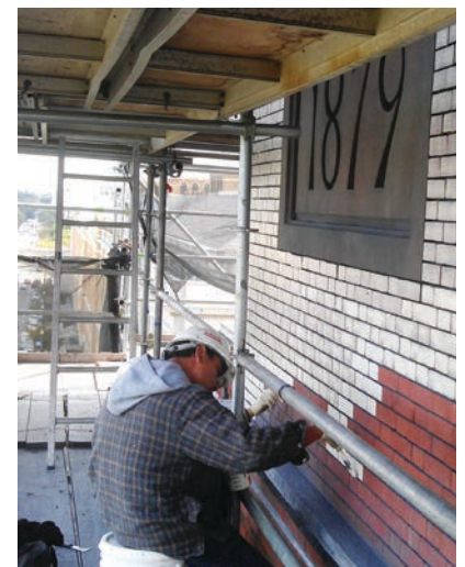
Sidney Yates Building Masonry Repointing & Exterior Repairs, Washington, DC
