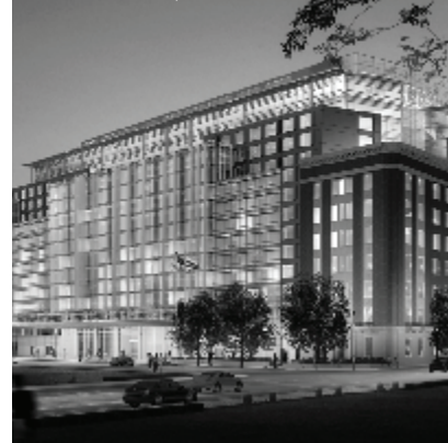
Marriott Marquis Hotel, Washington, DC Scheduled for Completion 2014
