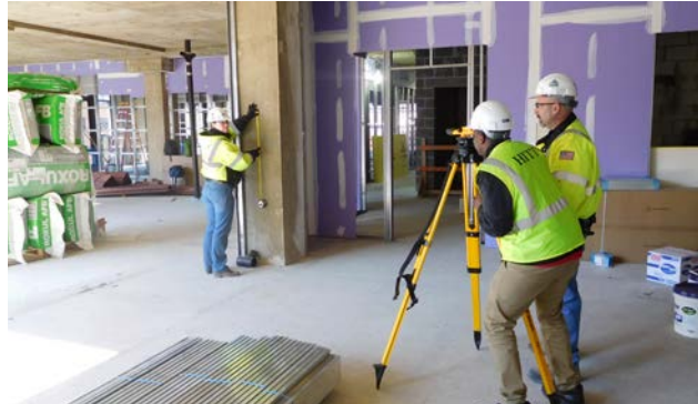
HITT Contracting, Inc
