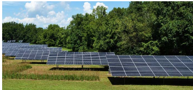
Ground: if an owner has the space can offset the majority of an owners kWh consumption, 600,000 plus per year for this farm:
