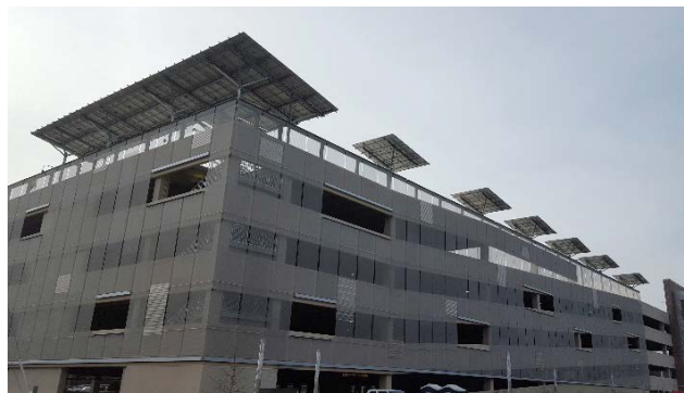
Carport: as shown for this university which offsets the entire load of the garage:
