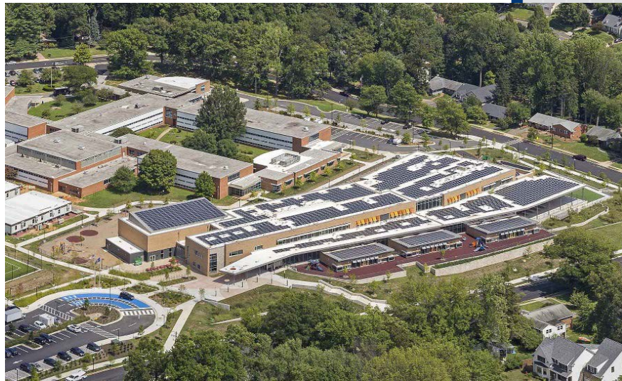
Roofs: flat with minimal obstructions or pitched toward the south, east, or west are ideal as shown for the new Net-Zero Williamsburg Elementary School in Arlington, VA:
