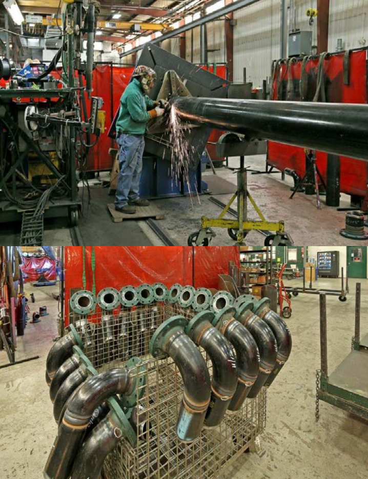
(Top) Steel shop pre-cutting pipe to length before it is released to the job site. (Bottom) Quantity of pre-fabricated pipe fittings.
