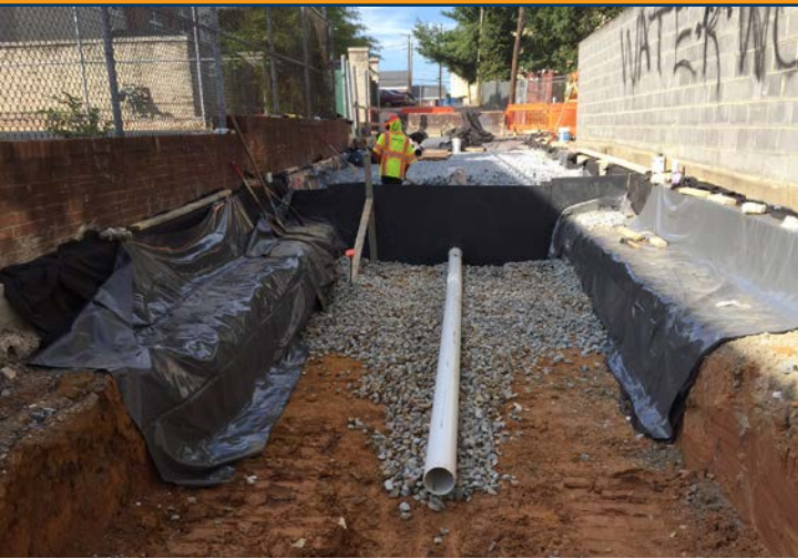
Perforated underdrain pipe, double-washed aggregate, and waterproofing liner (at sides) being installed by Anchor Construction as part of a permeable pavement facility in an alley.
