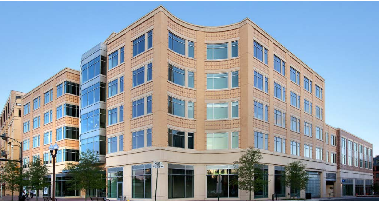
1776 full building from street.
