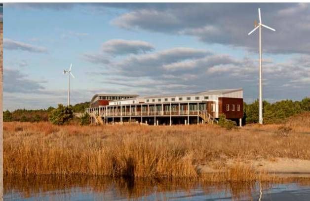
Credit: Hourigan Construction
