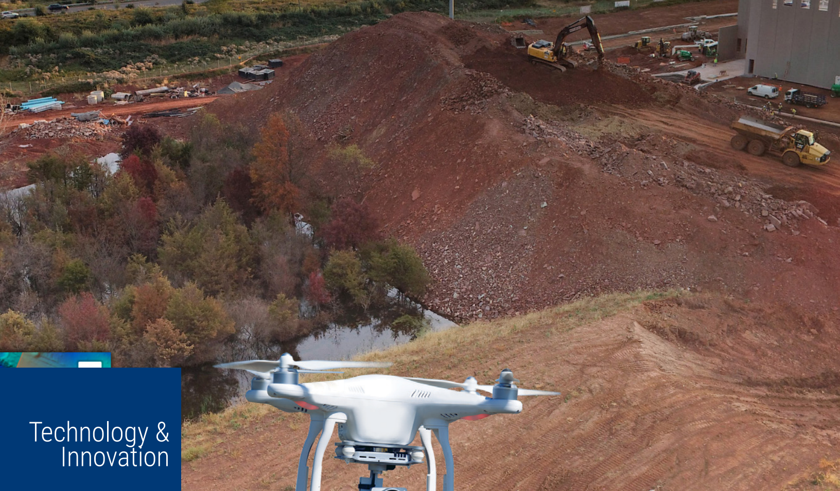
360 Imagery, Courtesy Hangar Jobsight
