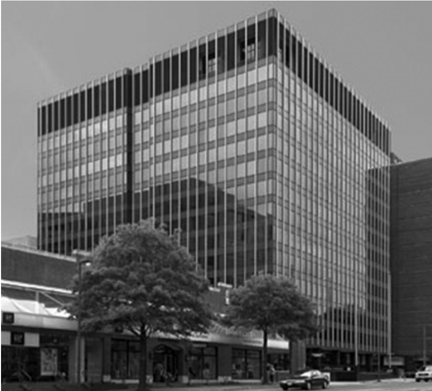
GPI Awarded Barlow Building Electrical Infrastructure Systems Replacement.
