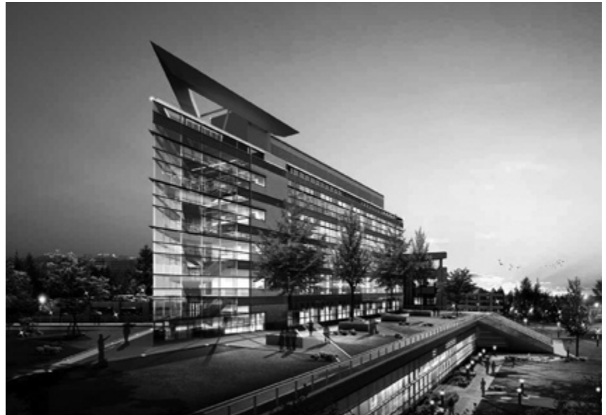
Army National Guard Readiness Center Addition (ARNG), Arlington, Va.
