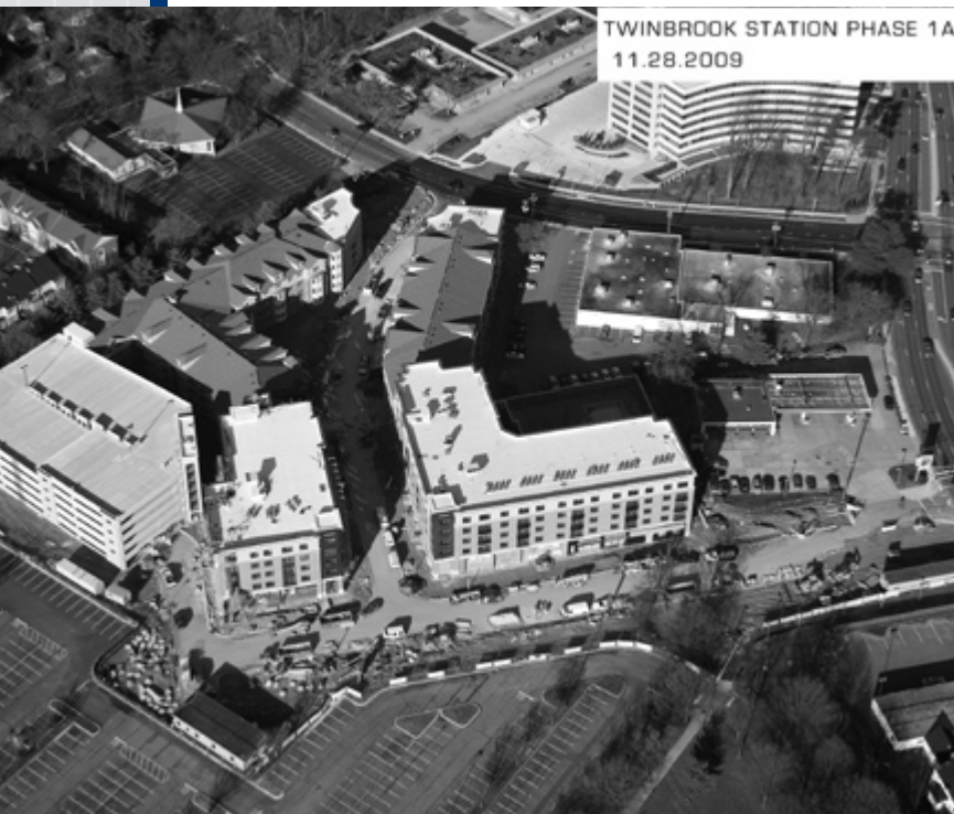
The Alaire under construction.
