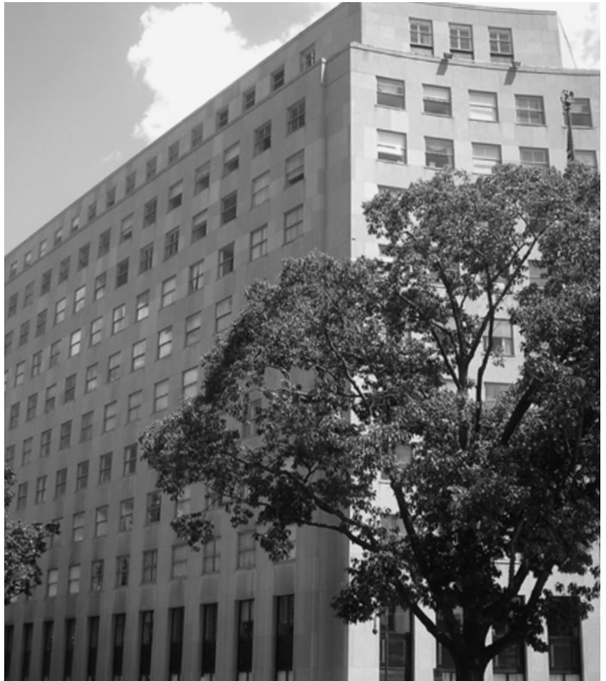
Grunley Construction will renovate the Lafayette Building in Washington, DC.
