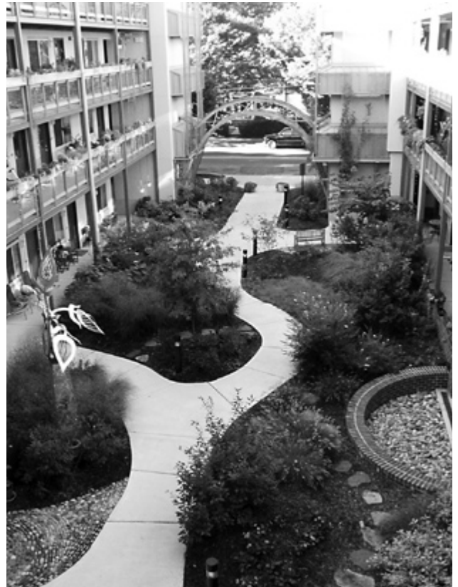
Eastern Village Cohousing in Silver Spring, MD is one of the first residential buildings in the U.S. to attain a LEED Silver rating for environmental performance.
